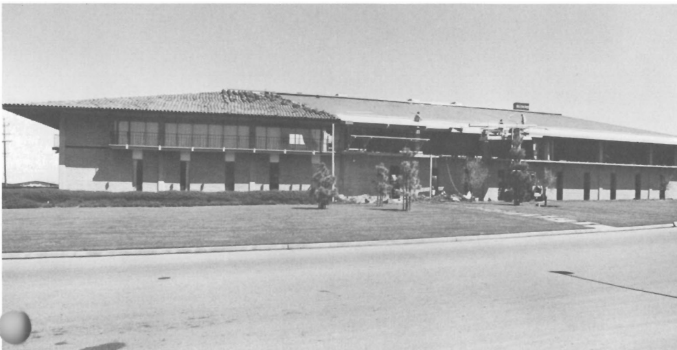
Until a few months ago this International Operations headquarters in Stanford Industrial Park represented the first half of a total building design. It was purchased that way in November, 1967 from a publishing company. Now the design is being carried out to its full size of some 25,000 square feet, to provide much needed space for International's global growth.
